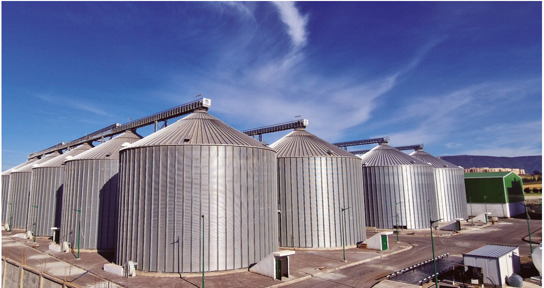
Plant in Annaba, Algeria. 1,000 t of steel were used to build the 100,000 t cereal storage plant.
