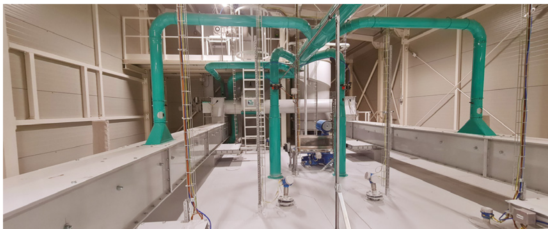
Supply and installation of a complete silo loading system (Defino & Giancaspro).
